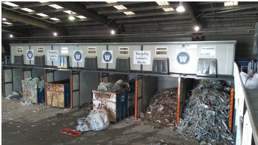
Figure 1 – Existing Picking Station at Maybank Wharf
